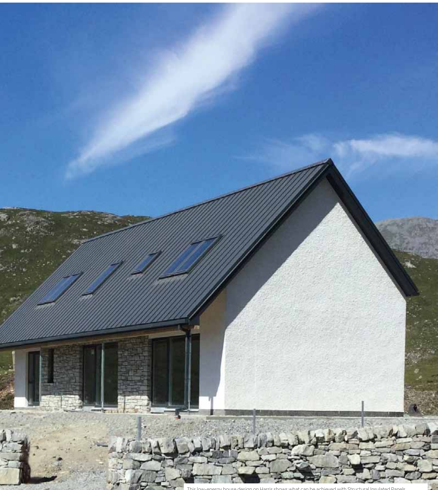
This low-energy house design on Harris shows what can be achieved with Structural Insulated Panels
