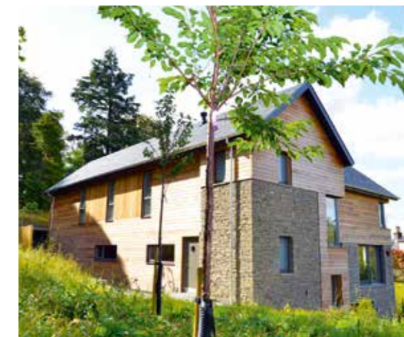
Left: Horizontally and vertically laid cladding was paired with a stone to complete this house, which was built by JML Contracts
