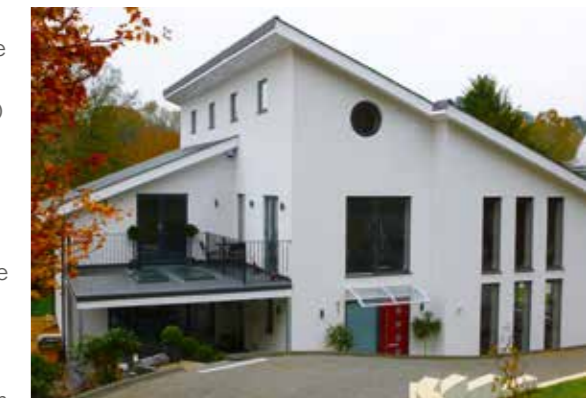
Above: Built by Eco SIPs Homes, this dwelling's asymmetric form and crisp rendered finish give it a striking look
