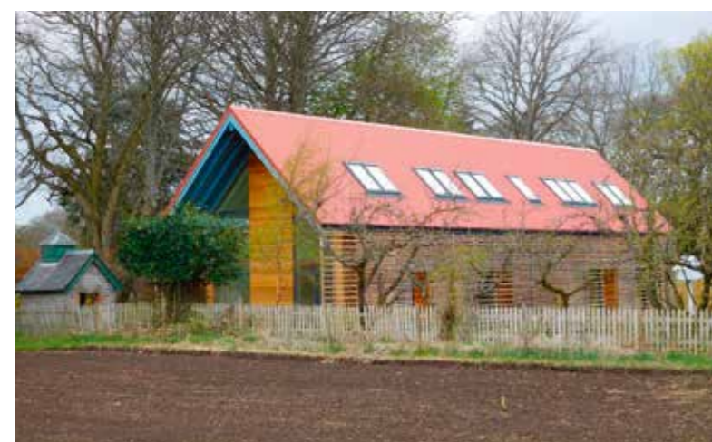
Above: A barn-style SIPs house by Model D Homes. Large swathes of glazing and horizontally-laid cladding give the building a modern look
