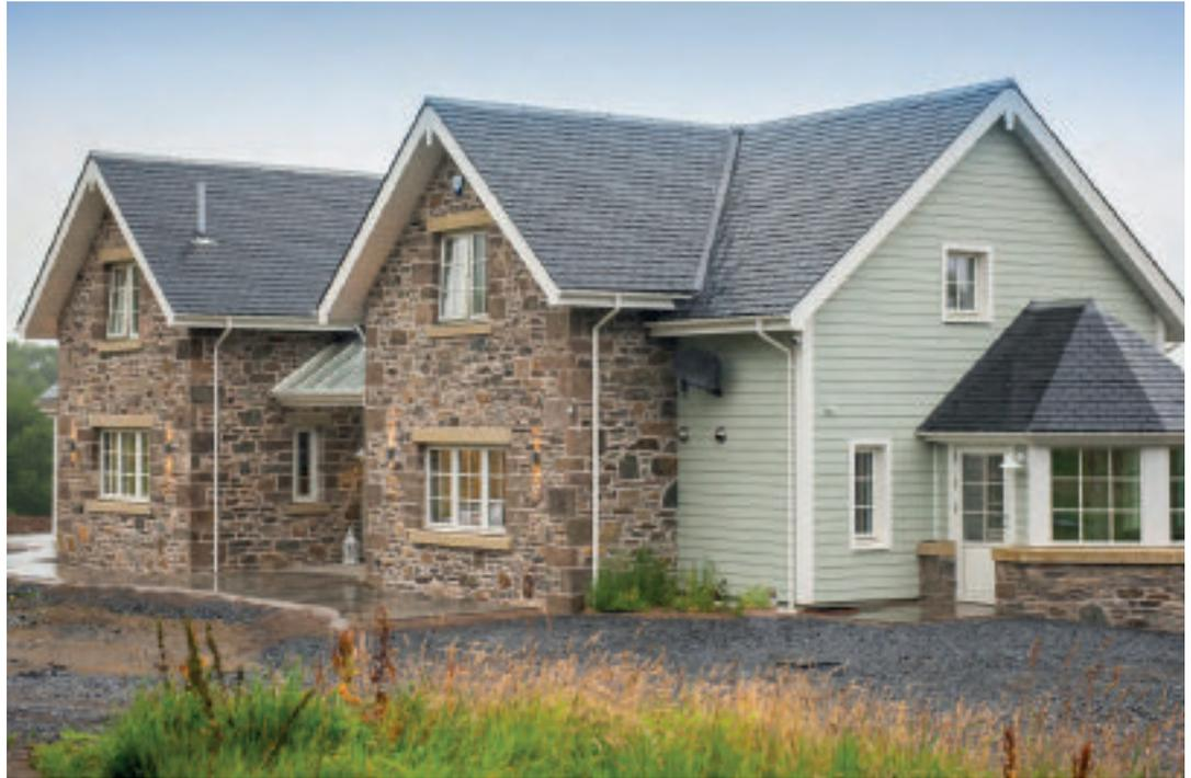
winter and overheating in the summer months. By using SIPs combined with a mechanical ventilation system, we were able to ensure that David and Pia's home is thermally efficient all year round.
